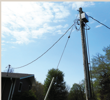
The power line running from the meter pole to serve a building is owned by the property owner, not the cooperative. That means co-op members also own any service disconnect and breakers that extend from the meter to their property. Your electric cooperative does not provide service or maintenance on this equipment.
